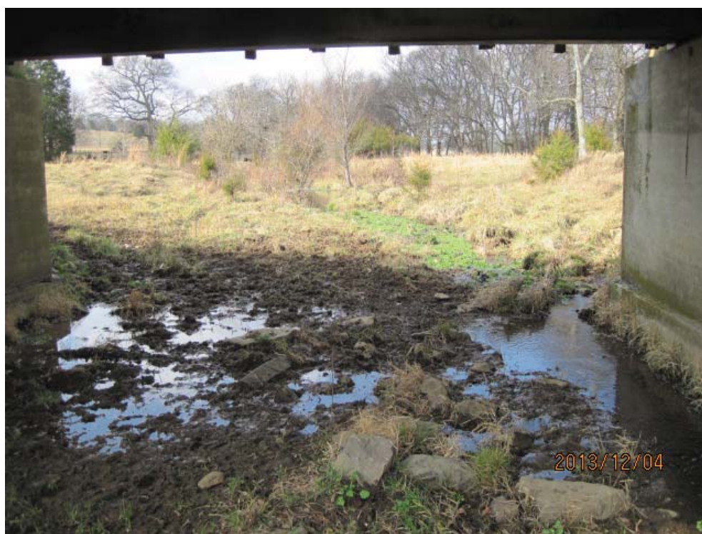
Photo 4: STR-2, branch @ LM 5.45 facing upstream
